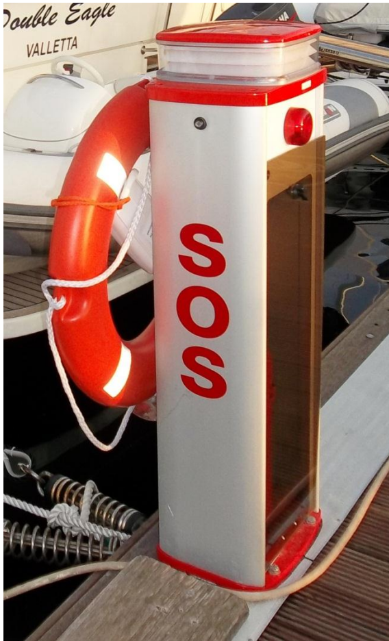
Figure 1. (above) The SOS Pedestals showing the life ring, red light, and fire extinguisher cabinets. Also contained in each cabinet is a fire blanket and first aid kit.
